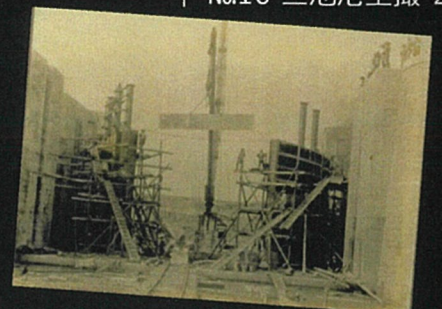
↑ No.1 閘門鐵扉組立
